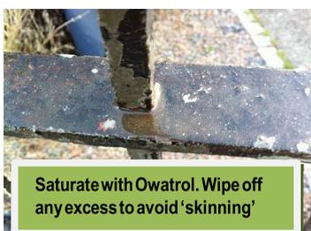
Using a 50mm approx. paint brush (or a spray device) saturate a section of the heavily scaled rust totally with Owatrol oil working from the top down.
