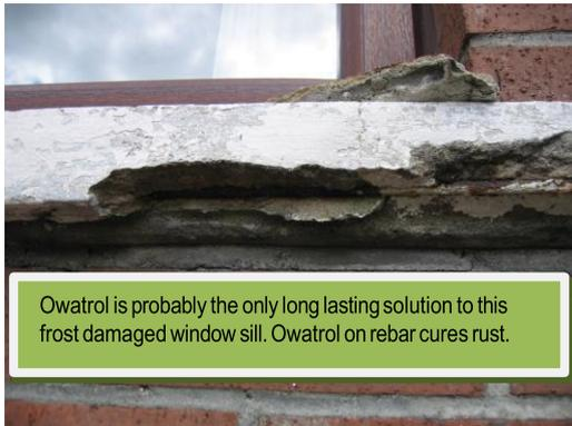
Sometimes you will encounter a concrete wall, sill, lintel etc. where water ingress and subsequent frost damage has caused the concrete to crack or even split into a crevice where you can even see the buried (rusted) steel reinforcing bar. Solution is as follows.
