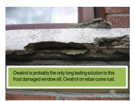
Sometimes you will encounter a concrete wall, sill, lintel etc. where water ingress and subsequent frost damage has caused the concrete to crack or even split into a crevice where you can even see the buried (rusted) steel reinforcing bar. Solution is as follows. If only a crack, feed Owatrol oil into the crack and allow to dry over a few days. That can be
