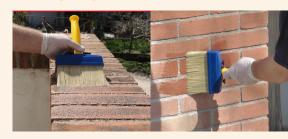
BKK is based on silanes and siloxanes which form a water-repellent matrix within the masonry. With a low molecular weight **BKK penetrate deeply** into the
