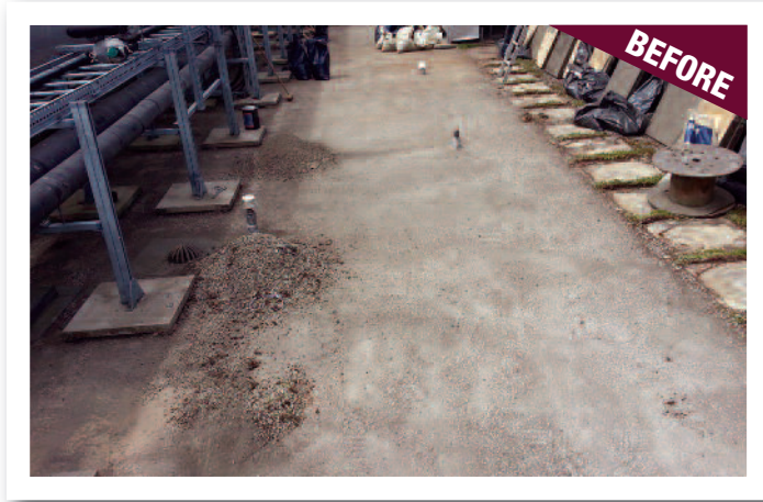
Scarborough Hospital, Asphalt Roof, Work begins
