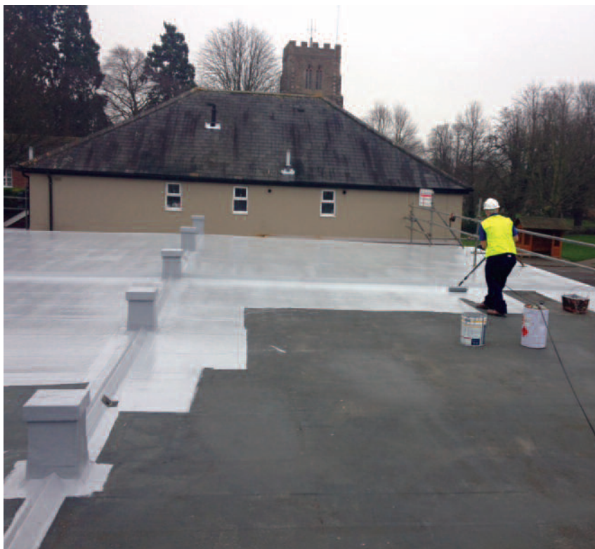
Seamless GacoPro being applied
