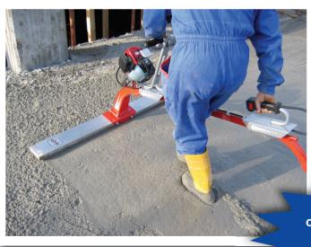
This wet screed or concrete levelling machine is a must have for any company or person / business working with concrete making floors, paths, driveways, paving, sites etc because it saves so much time and labour.
